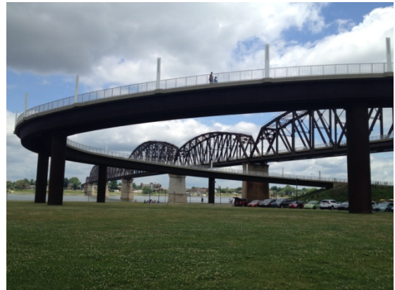
Big Four Bridge in Louisville, Kentucky Photo by KYTC, 2014
